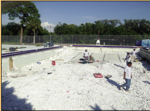
Pool Construction Update and Photos, Page 2
