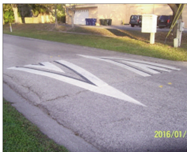
View of existing traffic calming looking south toward speed table.
