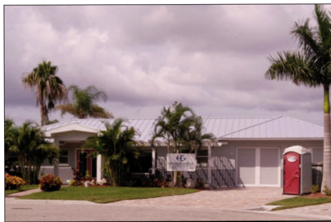
A new roof, plus a new two-car garage and big interior renos are just about complete at this Bayshore Gardens home on Bay Drive West.
